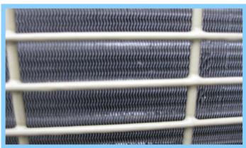
**Situation:** Galveston Island is one of the most corrosive areas in the country, due to continuous salt-spray intrusion and from the many chemical and oil refineries in the area. Typical uncoated or competitive product coated condenser coils would survive only 3 to 4 years before need of replacement.
